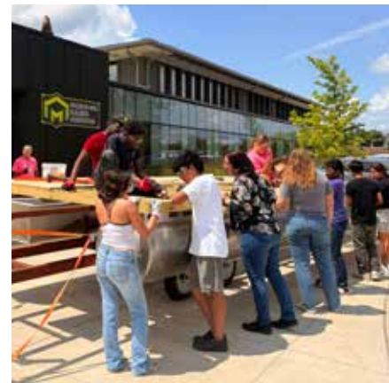
Campers building pontoon project for Mad City Ski team.
